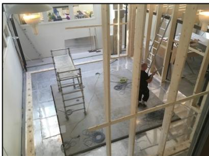
A new TEM will soon be installed in the Arrhenius laboratory at Stockholm University. The room where it will be placed are slowly appearing in the old chemistry library. The photo shows among others the concrete foundation, the aluminium sheets for the Faradays cage and cables for the field cancellation system. The delivering date for the instrument is planned to the beginning of June.
